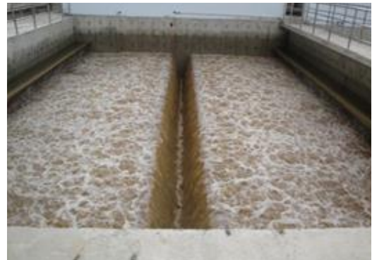
Filter in Backwash Mode
